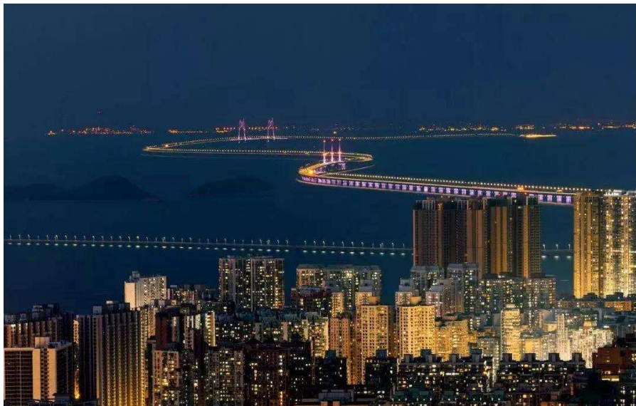
Hong Kong-Zhuhai-Macao Bridge the longest cross-sea bridge in the world
