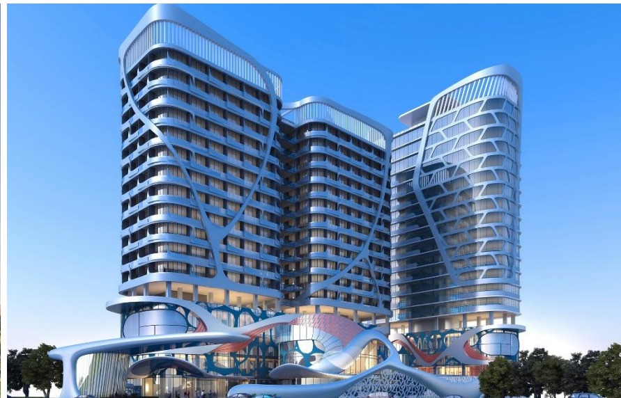
Prince IT Building, Cambodia
