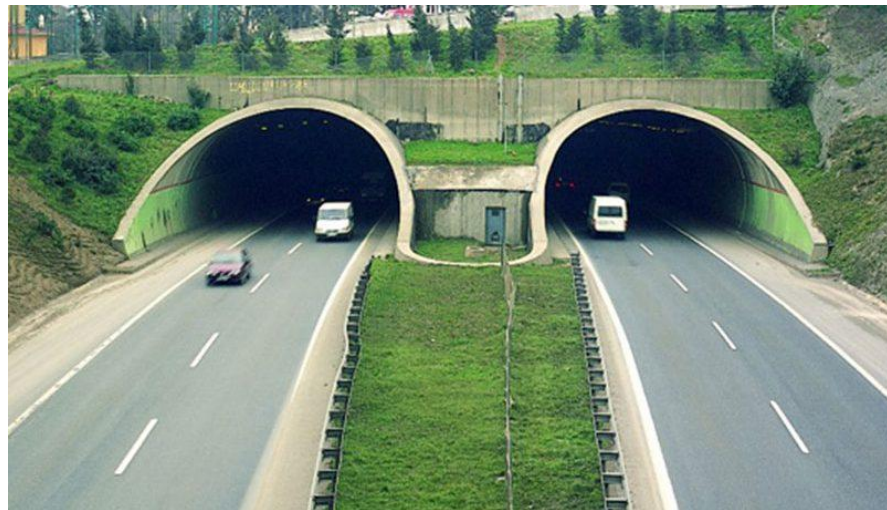
Chongqing Cimushan Tunnel
