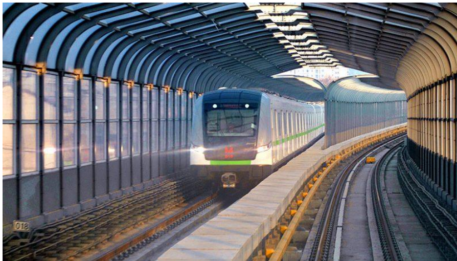
Phase II Project of Metro Line 4 of Wuhan
